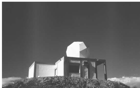
Fig. 1. The SST 3-m radome installed at CASLEO El Leoncito site
